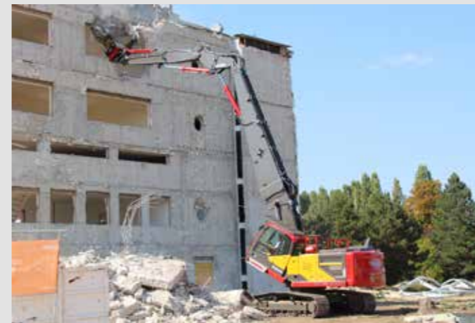
» Example 2 – High reach demolition front, Caterpillar 385
