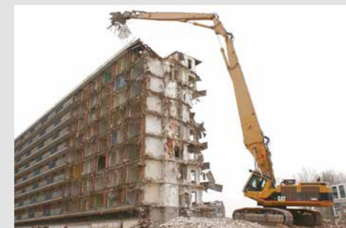
« Example 3 – Four piece high reach demolition front, ETEC 333
